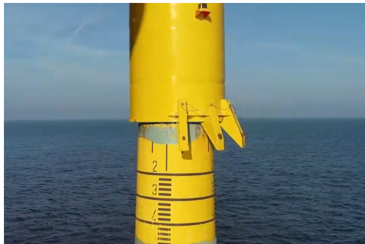
Figure 23 – Slip-joint connection
