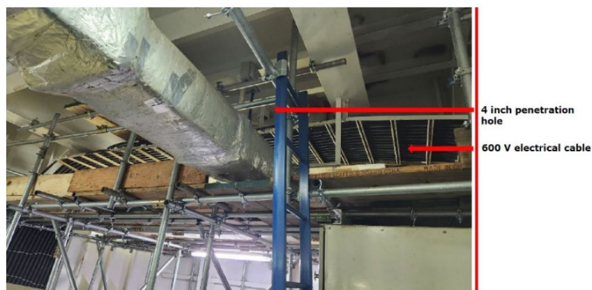
View from area below the deck
