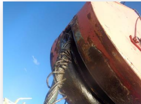
Figure 18 – Crane and rope failure
