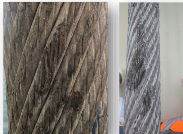
Figure 15 – Damage of the auxiliary hoist rope
