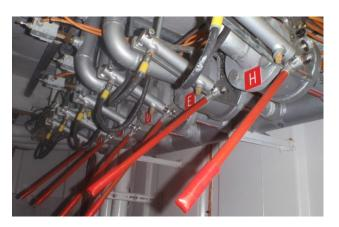
Hemp type pipe sealant was used extensively on pipe threads throughout the system and in some instances seems to have entered the system. (Photograph at right.)
