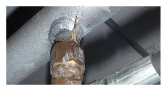
Certain elements of the distribution manifold contained low points which allowed the accumulation of water within piping that could not be drained. Such a circumstance could cause corrosion that could possibly negatively effect operation of other components. (Photographs at right.)
