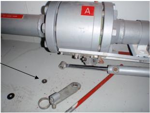
Actuating arms to five of the six other zone valves were found loose. They were also attached by small machine screws. (Photograph at right.)
